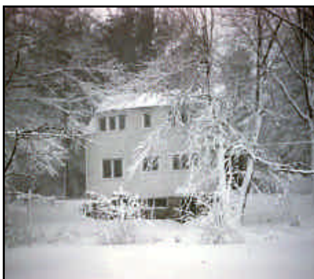
Quarters C pictured across Boundary Pond.
